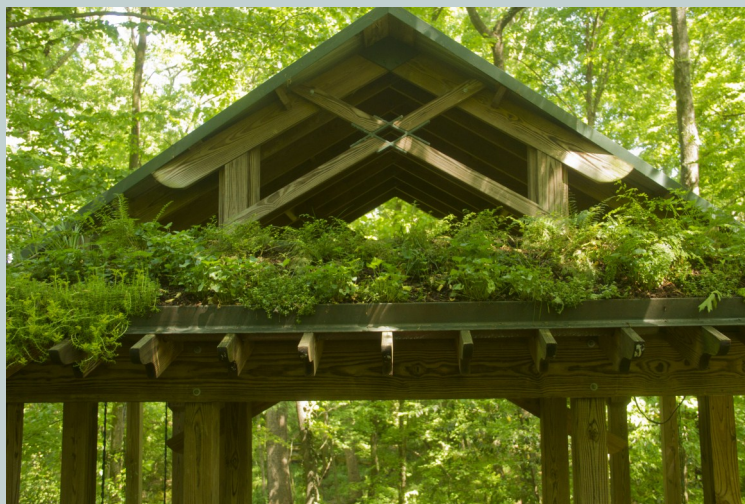
Green roof on outdoor pavilion
